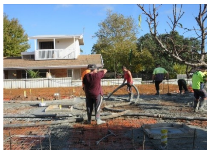
Pouring the concrete slabs
