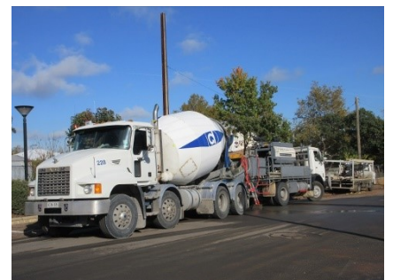
The concrete arrives
