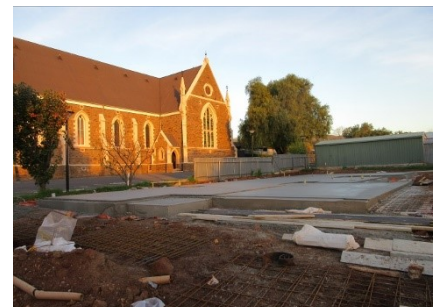
Slabs complete and curing
