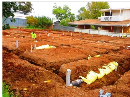
Drainage almost in place
