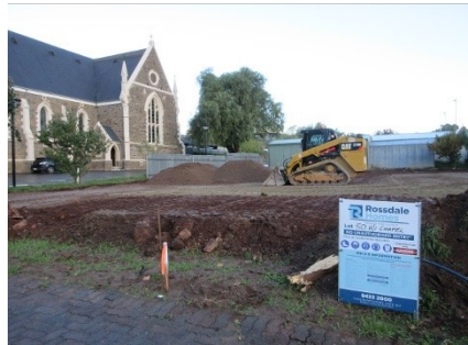
Levelling the ground
